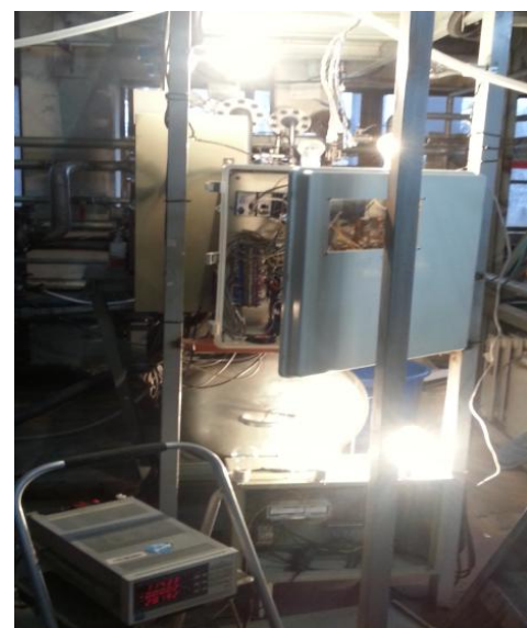
Figure 3: System under operation
