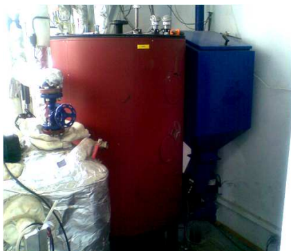
Figure 4: Prototype multi-fuel boiler with a solid fuel reservoir (biomass-pellets)
