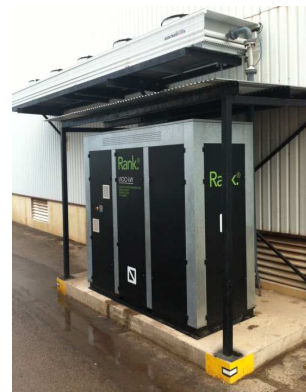
Figure 4: ORC modules: (a) Power generation system integrated in the industrial application, (b) CHP system during tests, (c) Power only and CHP system during tests.
